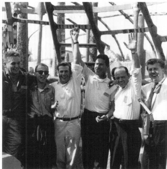
Photo taken by Seymour Rosen, 1959, just after the successful stress test that saved Watts Towers. Bud Goldstone is second from the left, in the dark glasses.
