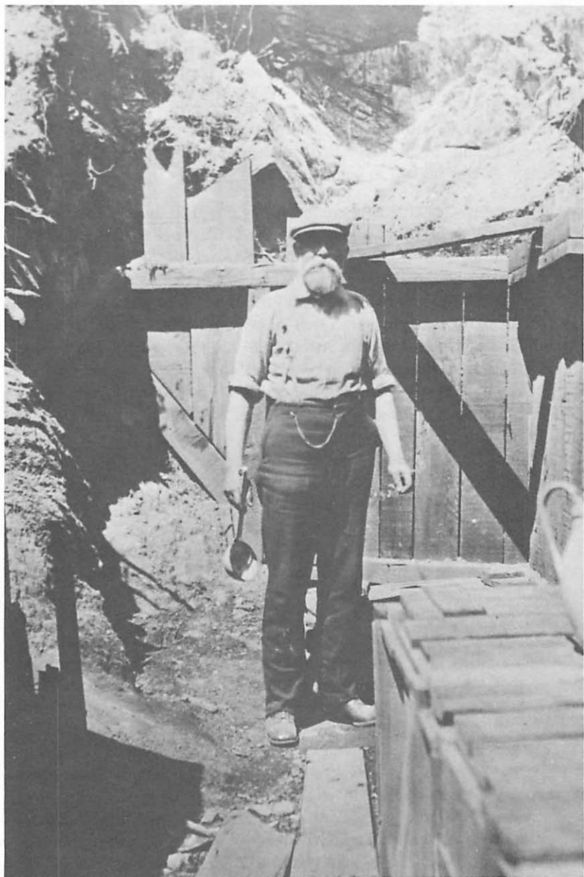
Hill at the Ingomar Consolidated Gold Mining Company in Calaveras County, California. The mine proved to be a financial loss for the Hill family.
