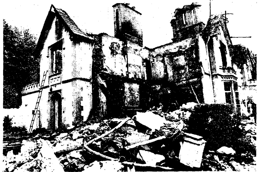
The remains of the house of Ivan Neill, Stormont speaker, destroyed by I.R.A.
