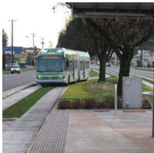
Figure 11 EmX Guideway and Station (Source: Lane Transit District)
