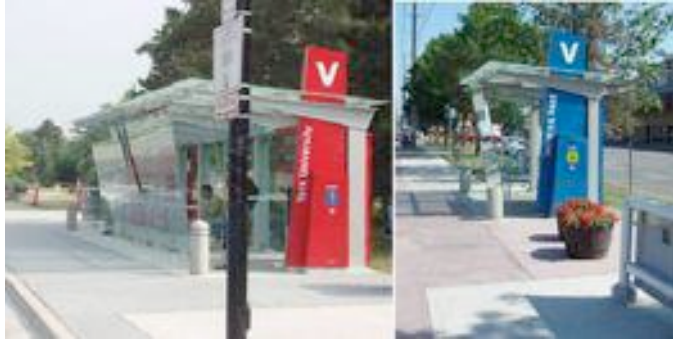
Figure 3 Station Stop Shelters for Viva (Source: York Region Transit)
