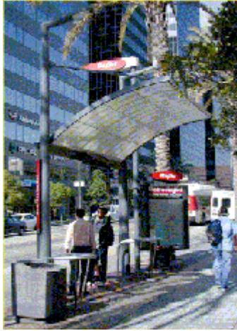
Figure 18 Metro Rapid Station
