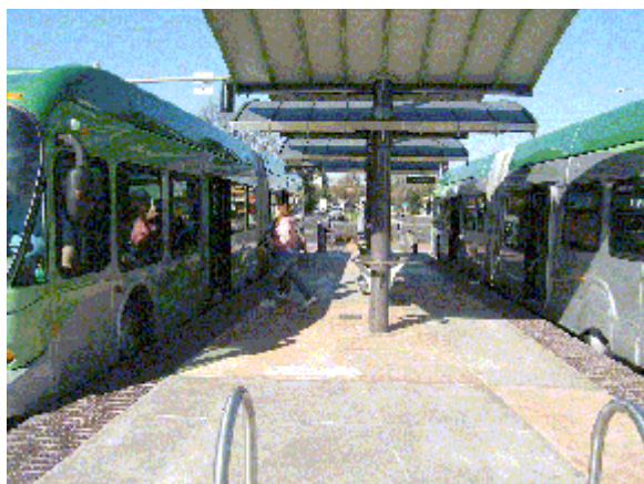
Figure 12 EmX Median Station Illustrating Left Side Bus Doors (Source: Lane Transit District)
