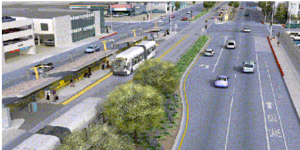
Figure 16 Orange Line Station (Source: Los Angeles County Metro)
