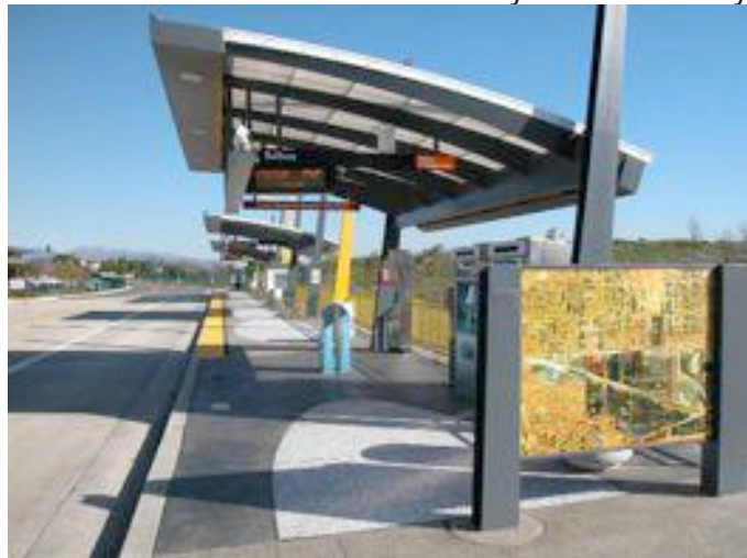
Figure 17 Orange Line Station Shelter (Source: Los Angeles County Metro)
