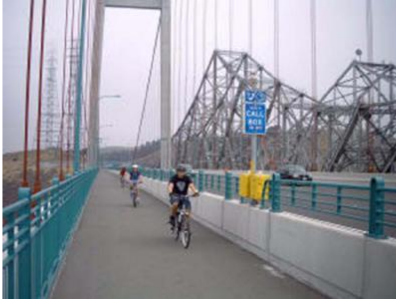
Figure 11 Carquinez Bridge bike lane
