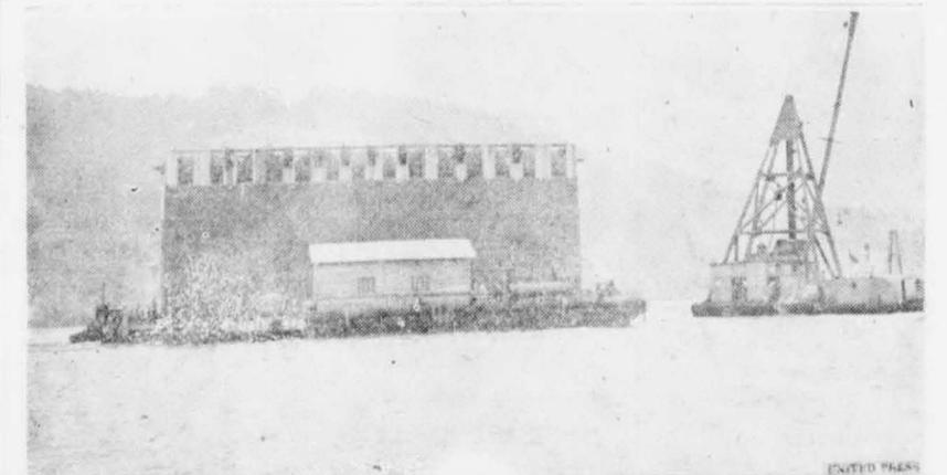
The steel and timber structure (pictured above) recently was towed into San Francisco by 1100 feet west of Yerba Buena island, where it will become the western end of one of the two 2310-foot suspension spans of the Oakland-San Francisco bay bridge. The huge caisson will be sunk to rock 170 feet below the water line and its steel cylinders, each 15 feet in diameter, filled with concrete.
