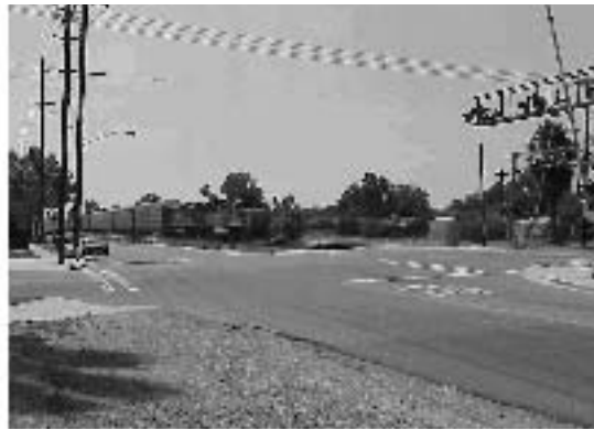
Figure 13. Railroad Crossing Mentioned as a Liability
