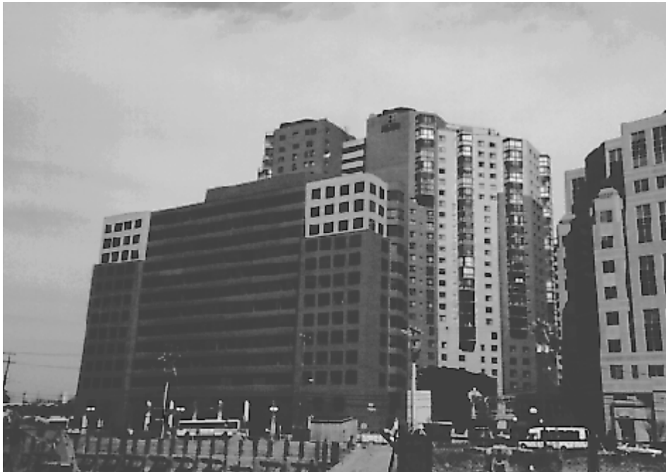
Figure 7-2 Another view of Ballston Metro Center
