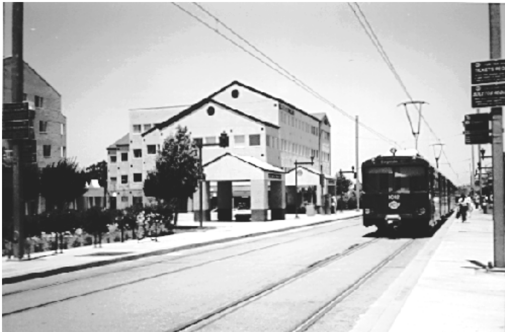
Figure 5-4 View of trolley station at La Mesa Village Plaza
