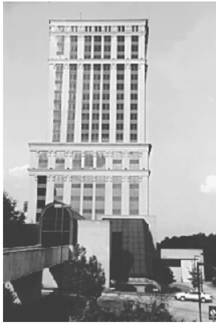
Figure 9-1 MARTA tunnel and Resurgens Plaza, Atlanta, GA
