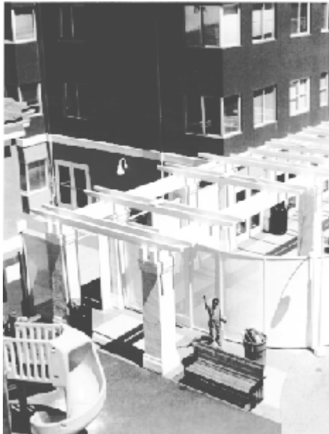
Figure 1-4 View of Play Area and Building A of Plaza Del Sol
