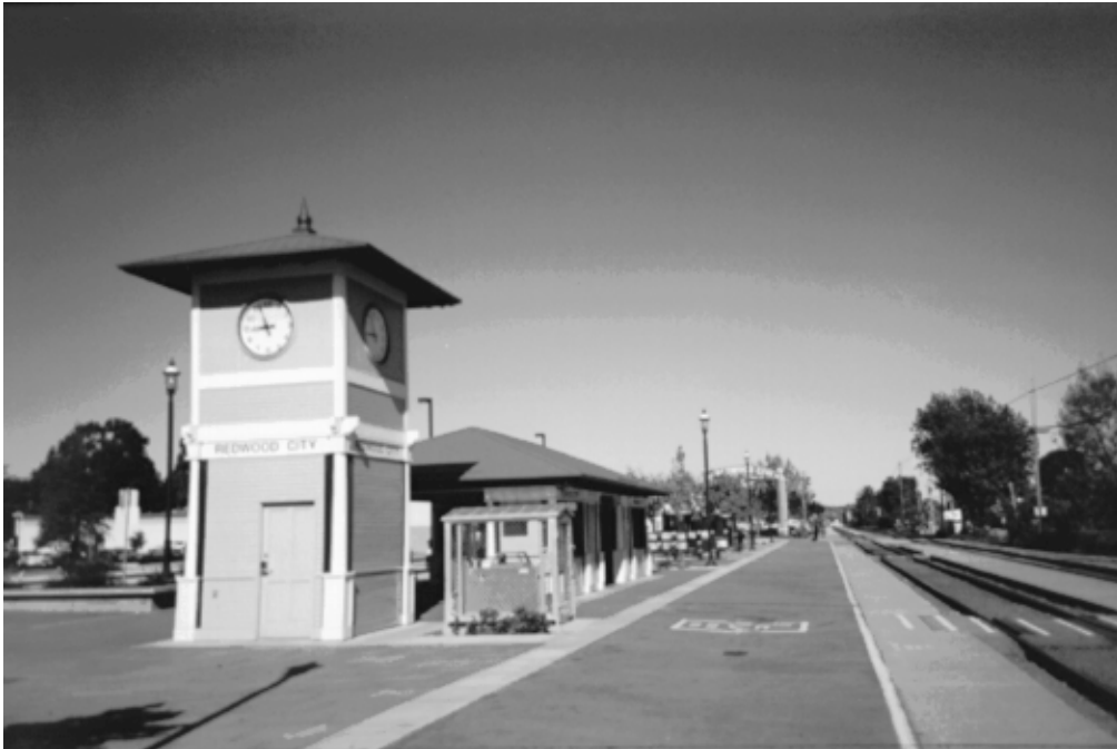
Figure 4-3 CalTrain depot in Redwood City
