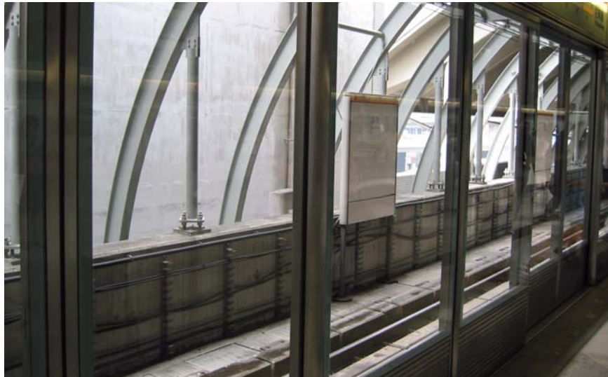
Figure 16 Another View of Platform Edge Doors, Hong Kong
