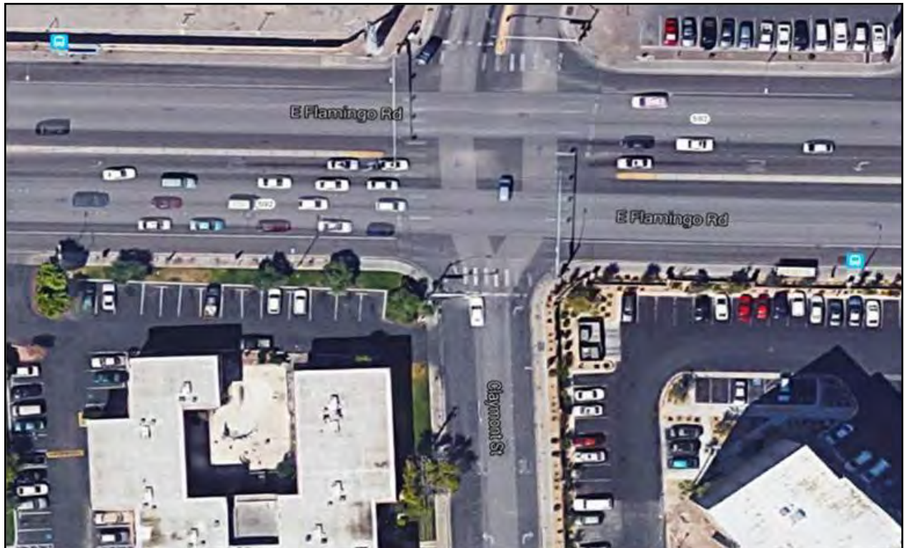
Figure 17. Possible Locations for a Bikesharing Station at Flamingo Road and Claymont Street
