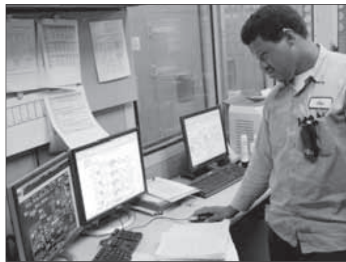
Otis Mcinnis, power plant operator for Facilities Development and Operations, demonstrates the computer system used to control and monitor the heating and cooling system that serves the entire campus on Monday. KEVIN HUME / SPARTAN DAILY
