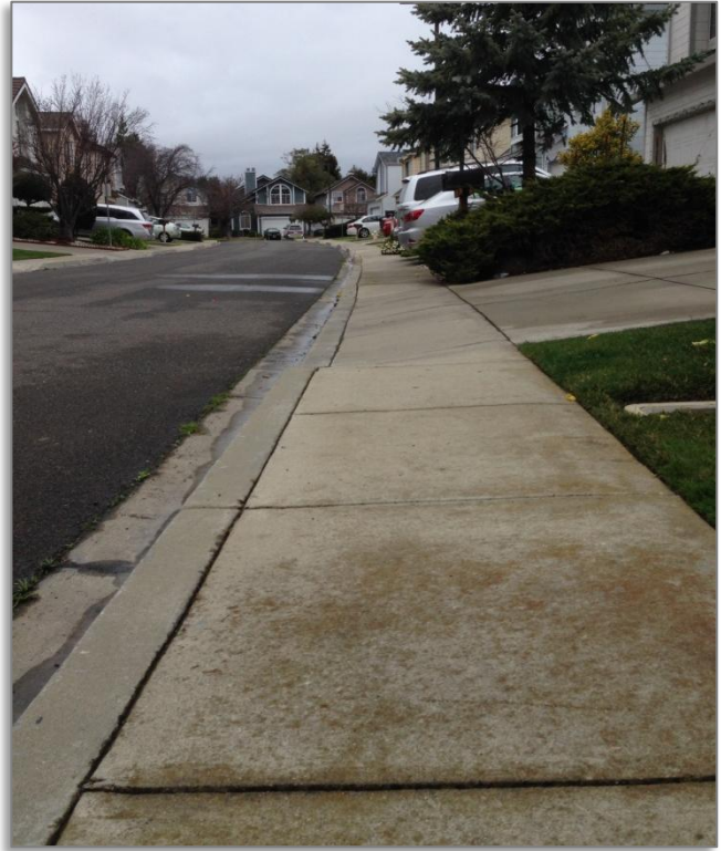
Figure 15. Four-foot sidewalk on residential segment. Even newer residential areas like this one near 34252 Xanadu Ter do not have the recommended 5-foot sidewalks. (Photo by Brish Miller, February 8, 2014)
