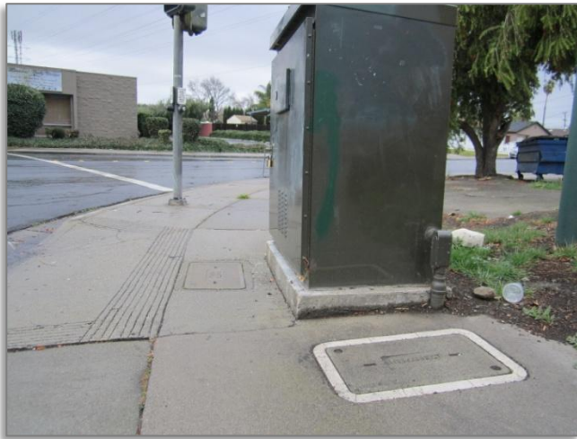
Figure 14. Obstruction due to traffic signal control cabinet. Obstructions like this one near 40675 Grimmer Blvd are particularly common at crosswalks in commercial areas. (Photo by author, February 2, 2014)
