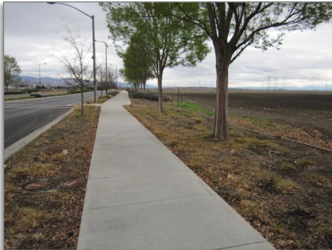
Figure 16. Immaculate new sidewalk in industrial area.
