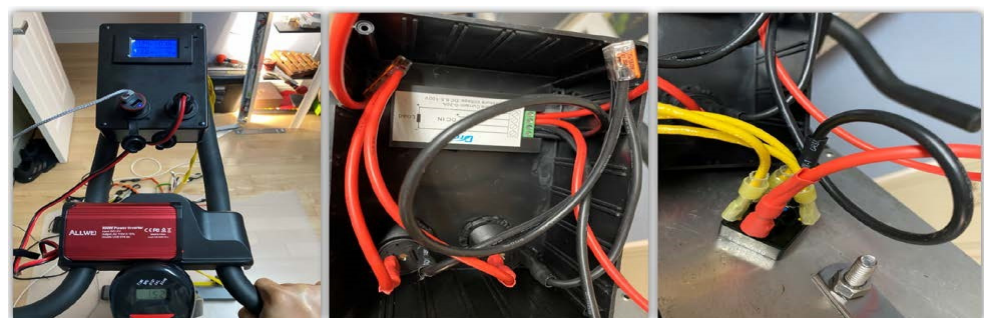
Figure 10. The electrical components on the prototype.
