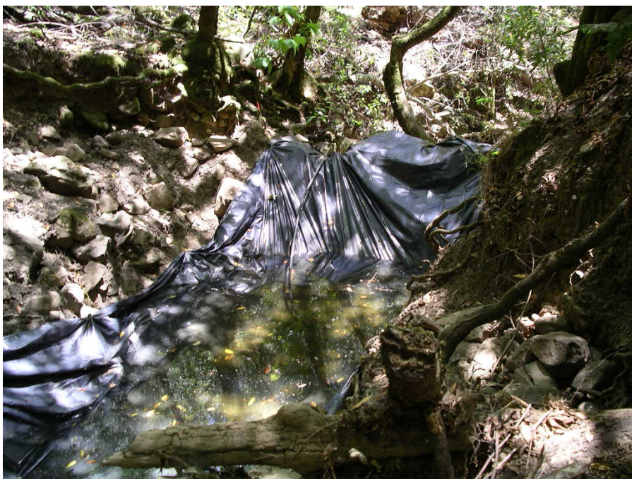
PHOTO 24.—Diversion dam that was constructed in a small perennial plunge pool on the tributary below Sheep Ridge. Irrigation lines brought water to the gardens downstream.
