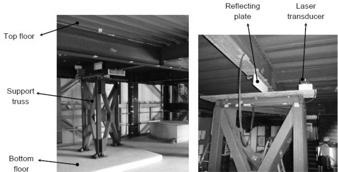
Figure 4.5. Laser Transducer and Reflecting Plate Instrumentation Mounted on Support Truss used for Measuring Inter-Story Drift (Ryan, n.d.)
