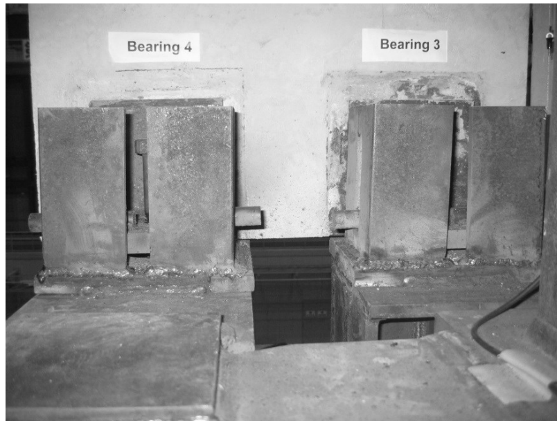
Figure 4.2. Bearing Connections at Base of 4th Floor (Photo credit: Maggie Ortiz, 2011)
