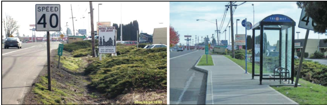
SW Oak & 17th – Before (Left) and After (Right) for Line 57-TV Highway Improvement, TriMet, Portland, Oregon
